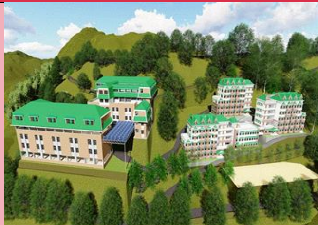
*HPNLU, Ghandal, Shimla, Building Complex under Construction.
